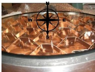
Once in place, fix the glass daylight collector into position with the three screws supplied through the steel ring and into the roof flashing. If we were informed of the desired system length in advance, the ceiling diffuser would have been provided pre-assembled to the tubing, therefore in this case the installation is now complete.
